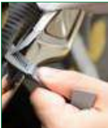
Press into the difficult corners. Insert your knife into the slot and cut.
